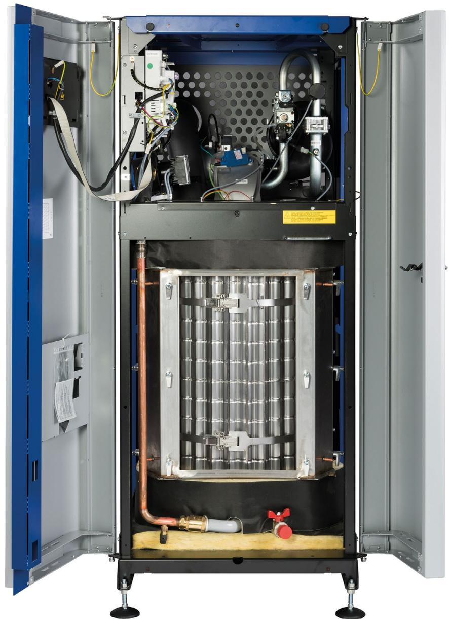
boiler, the internal circulation loop flow rate is modulated on a reducing basis to ensure high levels of system efficiency.
