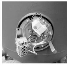
4 – Fit the heating element (thermostat at the top) and criss-cross tighten the assembly using the 6 M8 nuts. Tightening torque: 8 Nm
