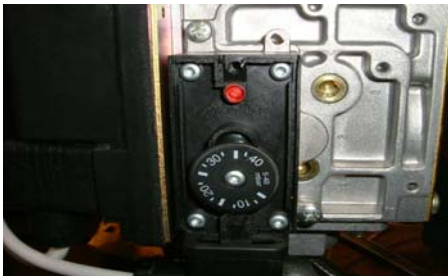
Fig 7.3.2 - Low Gas Inlet Pressure Switch
