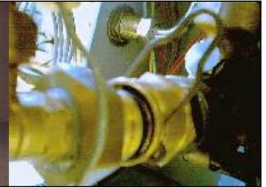
The power lead from the pump is connected to the mains terminal on the back wall of the unit. The connections are shown in Figure 24 below.
