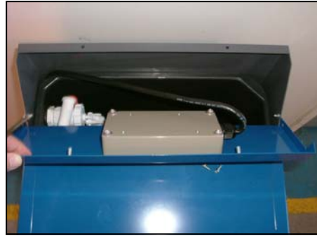
Figure 28 - Removal Of Inclined Panel
