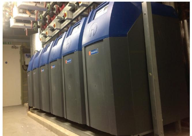
The Purewell Variheat condensing boilers have reduced **gas consumption by nearly 50%**. They provide the heating for the busy theatre as well as being the indirect primary heat source for the hot water via a Powerstock calorifier.
