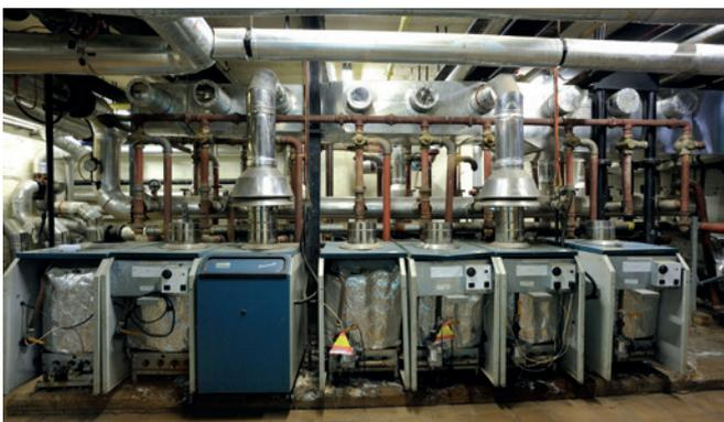
With older plant rooms access can inevitably be one of the main issues. The stairs to the Carlton Hotel's basement plant room are fairly steep and required the use of a crane to lift out the old boilers and install the new ones. Disassembled when access is problematic.
