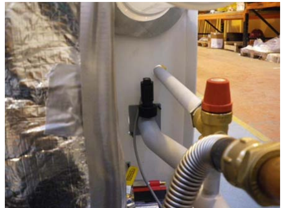
Figure 9.2 - Water Flow Switch
