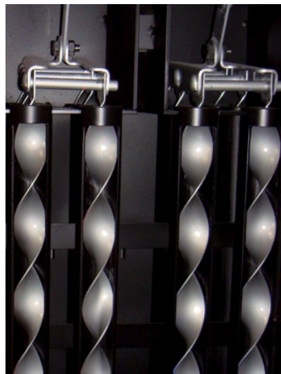
Helical turbulators
