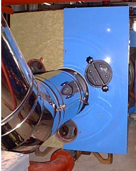
Picture 3: RH Rear Casing Fitted
