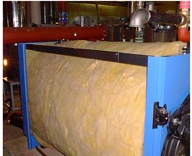
Picture 6: Side Rail attachment.
