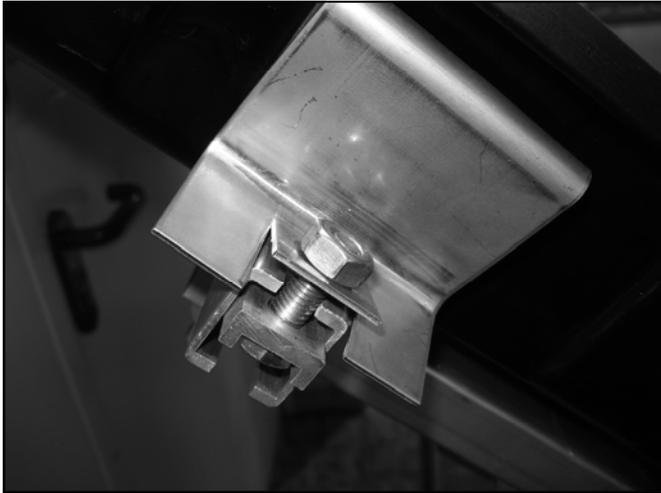
Figure 13.4.18 Assembly Of Single Attachment Clamp
