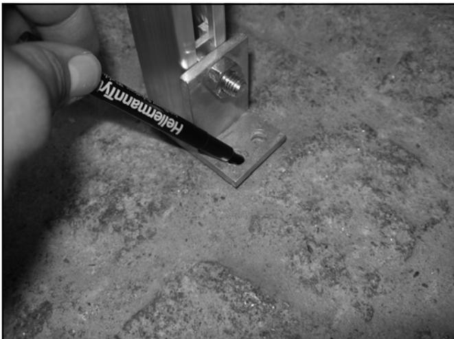
Figure 13.4.19—Marking The Foot Bracket Holes
