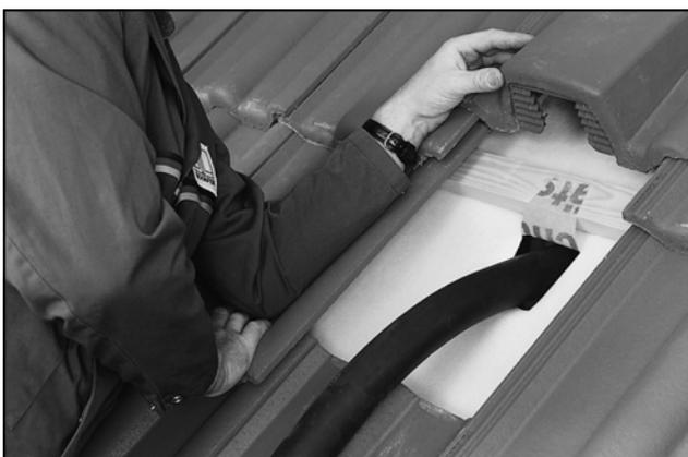
Figure 12.18 - Tube Entry Into Roof Space
