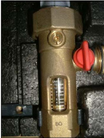
Figure 15.11 Flowmeter Setting Valve
