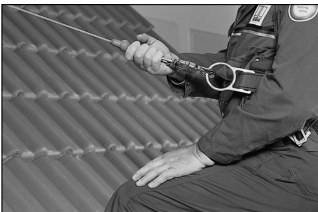
Figure 14.3 - Always Wear A Safety Harness and use a safety line.
