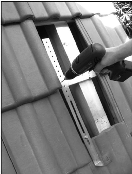
Figure 12.6 - Assembly Of Attachment Anchor Bracket.
