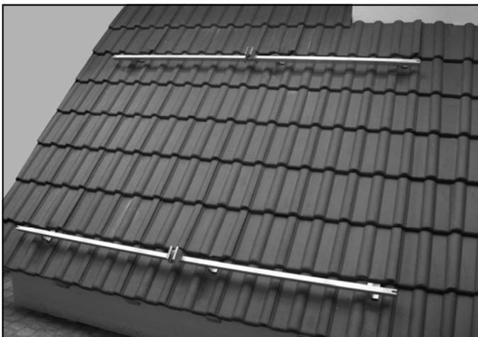
Figure 12.9 Assembly Of Upper & Lower Rails On Roof
