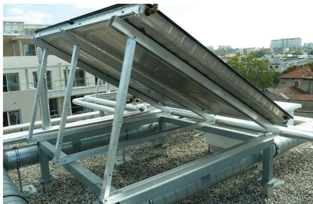
Trigon 2.3V collector array, flat roof mounted using a shallow A-Frame array fixing kit
