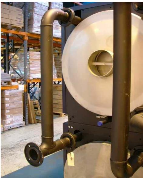
**10.3.3** - Using nuts and bolts supplied fit Warm Return Header (Item 3 on list, see page 15) as shown in figure 10.3.3, ensuring that correctly sized gaskets are in place.
