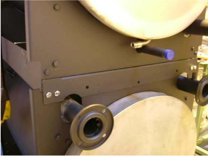
**10.1.9 - Ansty AD540 and AD640 Models only.** To fill gap between upper and lower boilers fit rear junction plate as indicated in figure 10.1.9.
