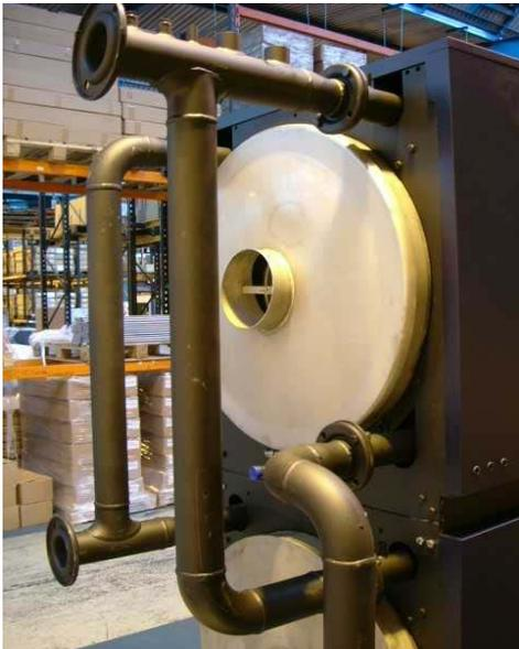
**10.3.2** - Using nuts and bolts supplied fit Flow Header (Item 1 on list, see page 15) as shown in figure 10.3.2, ensuring that correctly sized gaskets are in place.
