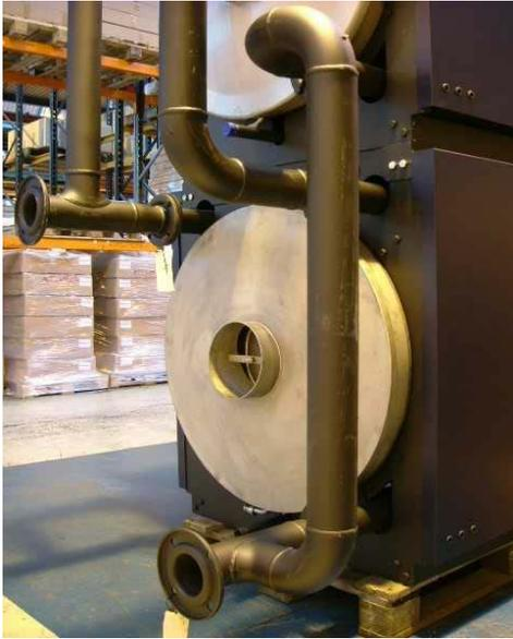
**10.3.1** - A box of fixings and gaskets for the pipework assembly kit can be found in the furnace of each boiler. Using nuts and bolts from this box, attach Cold Return Header (item 2 on list, see page 15) to pipe fittings on left hand side of boiler looking from the rear as shown in figure 10.3.1, ensuring that correctly sized gaskets are in place.
