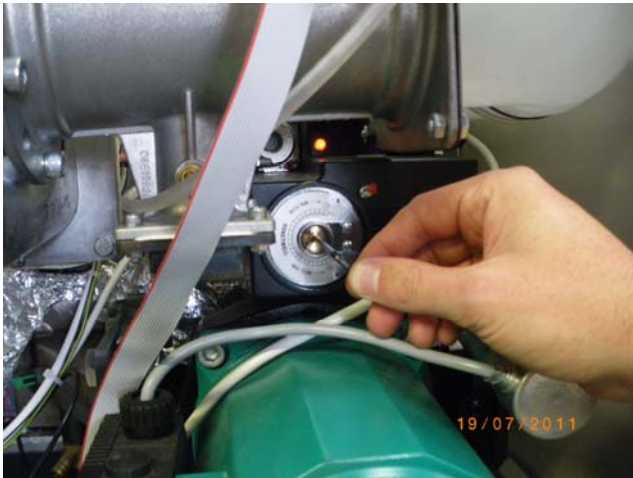
Figure 7.6.1- Adjusting gas valve throttle
