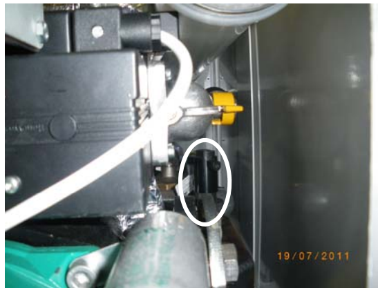
Figure 9.2 - Water Flow Switch
