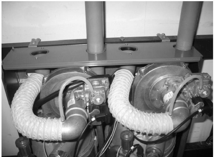
**Figure 5.2.1 - Twin Duct connection**
