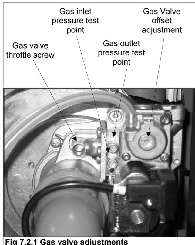
**Fig 7.2.1 Gas valve adjustments**
