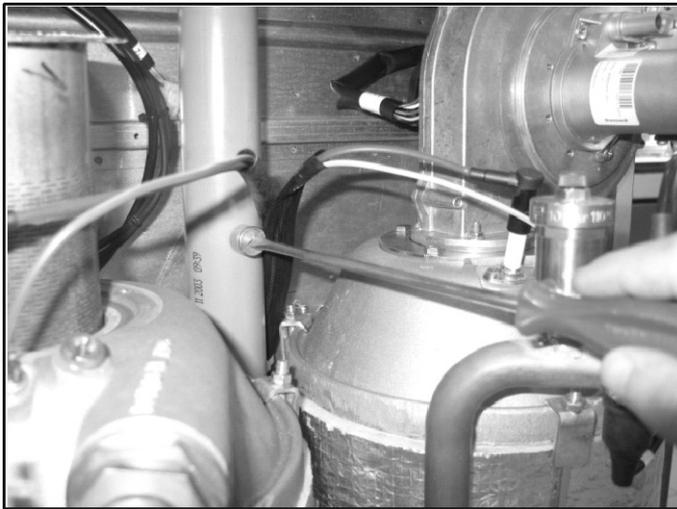
Fig 7.3.1 - Flue gas analysis point
