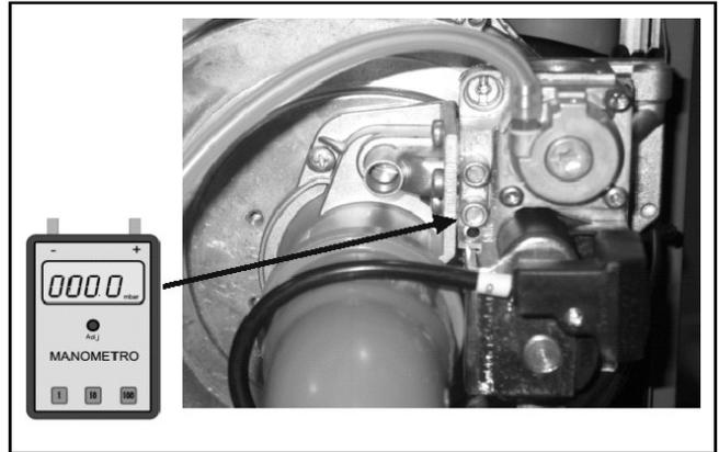
Fig 7.2.2 - Gas Inlet Pressure Test Point
