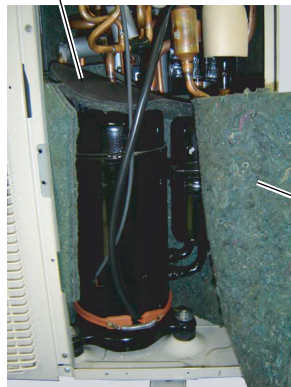
Remove the COMPRESSOR COVER A and TOP.
