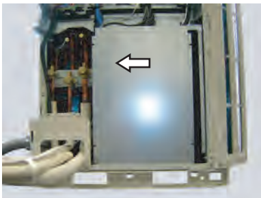
Remove the Comp box cover by sliding leftward and toward.
