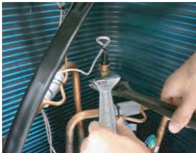
Remove the PRESSURE SENSOR with wrench.
