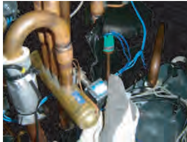
Remove the SOLENOID COIL.
