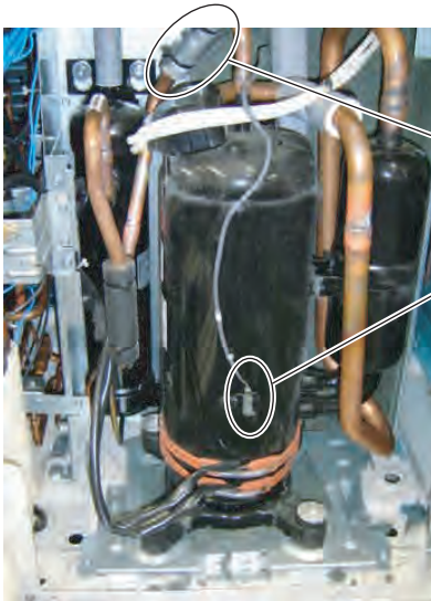
Discharge temp. thermistor (TH1)
