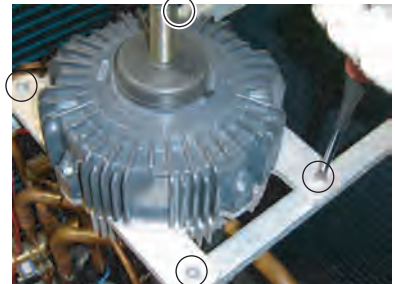
Remove the 4 mounting screws. Remove the Fan motor.
