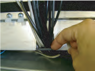
Remove the locking stopper of edging saddle.(3 places)
