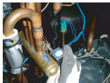
Remove the SOLENOID COIL.
