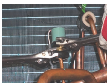
Remove the PRESSURE SENSOR with wrench. There are two sensors. (High and Low pressure)
