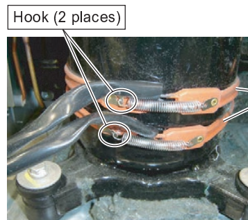
Crank Case Heater (2 places)
