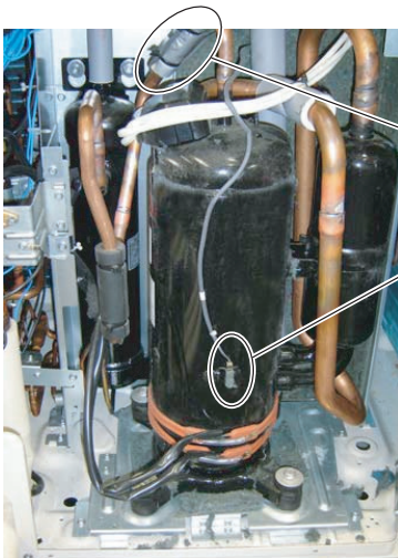
Discharge temp. thermistor (TH1)
