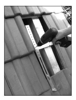
Figure 12.6 - Assembly Of Attachment Anchor Bracket.
