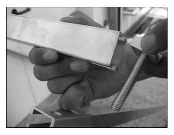
Figure 13.4.7 - Horizontal rail assembly
