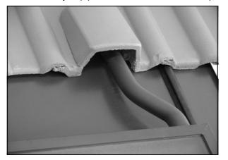
Figure 3.1 Example Of A Tile Type Roof Terminal
