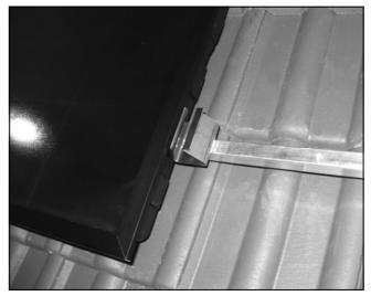
Figure 12.12— Collector Assembled To Rails
