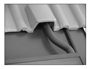
Figure 14.16—Tile Type Roof Terminal Assembly
