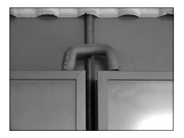
Figure 14.13—Assembly Of Connection Hose
