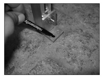
Figure 13.4.19—Marking The Foot Bracket Holes
