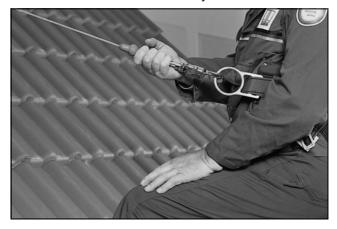
Figure 12.4 - Always Wear A Safety Harness and use a safety line.
