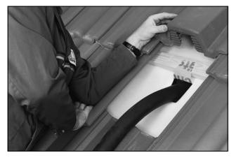
Figure 12.18 - Tube Entry Into Roof Space
