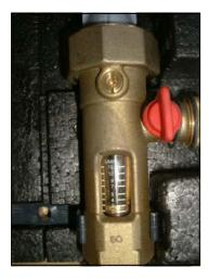
Figure 15.11 Flowmeter Setting Valve
