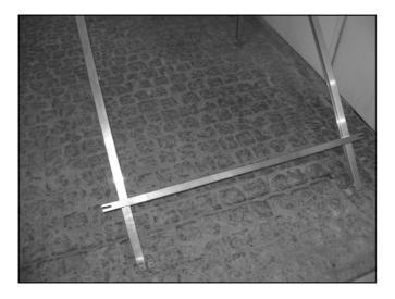
Figure 13.4.10 - Assembly Of Lower Horizontal Rail
