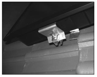
Figure 12.13-Outer Attachment Clamp Assembly Detail
