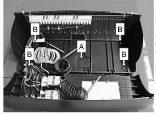
Remove the cable entry blanking plate (A) from the control console and screw the control panel to the top cover using the 4x10self tapping screws (B).
