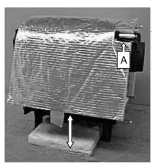
Wrap the insulation jacket around the boiler sections. Check that the cut outs (A) are positioned around the rear spacers and secure in position with duct tape.
