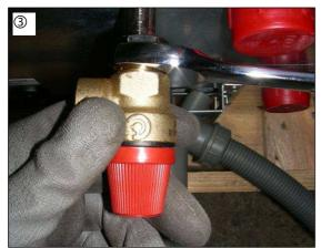
Securely hold the valve when tightening the nut to prevent any deformation of the tube.
