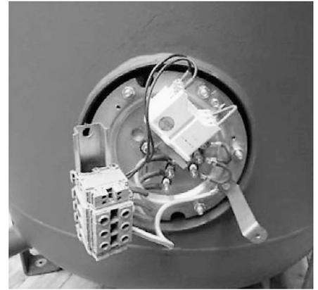
4 – Fit the heating element (**thermostat at the top**) and criss-cross tighten the assembly using the 6 M8 nuts. Tightening torque: 8 Nm
