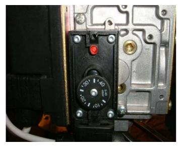
Figure 8.1.2 - Low Gas Inlet Pressure Switch
