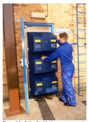
Figure 2.2 - Boiler Positioning
