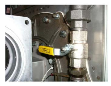
1. Ensure the boiler module gas service valve is closed (Figure 8.1.1)
