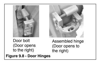
9.8.3 Lift the door in the open position and locate the hinges over the hinge pins. Carefully close the door and check that when the 4xM16 door locking bolts and washers are tightened the tongue on the front section closes firmly on the rope seal around the door. Open the door and check that there is an indentation in the rigid door insulation from the tongue on the front section around the combustion chamber hence illustrating a satisfactory seal.
