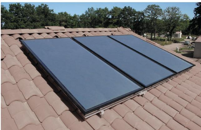
Single field array of three Trigon 2.3V vertical collectors, rail-mounted on a tiled sloping roof
