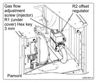
figure 44 - Gas valve models 180 to 450
