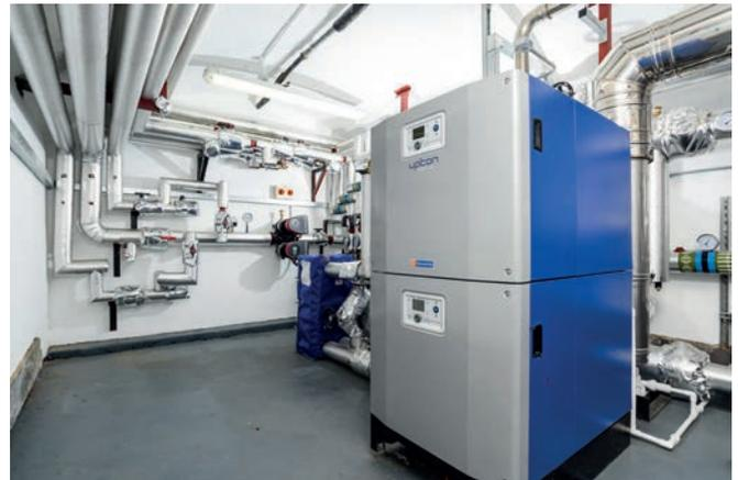
Upton boiler and plate heat exchanger (left).
