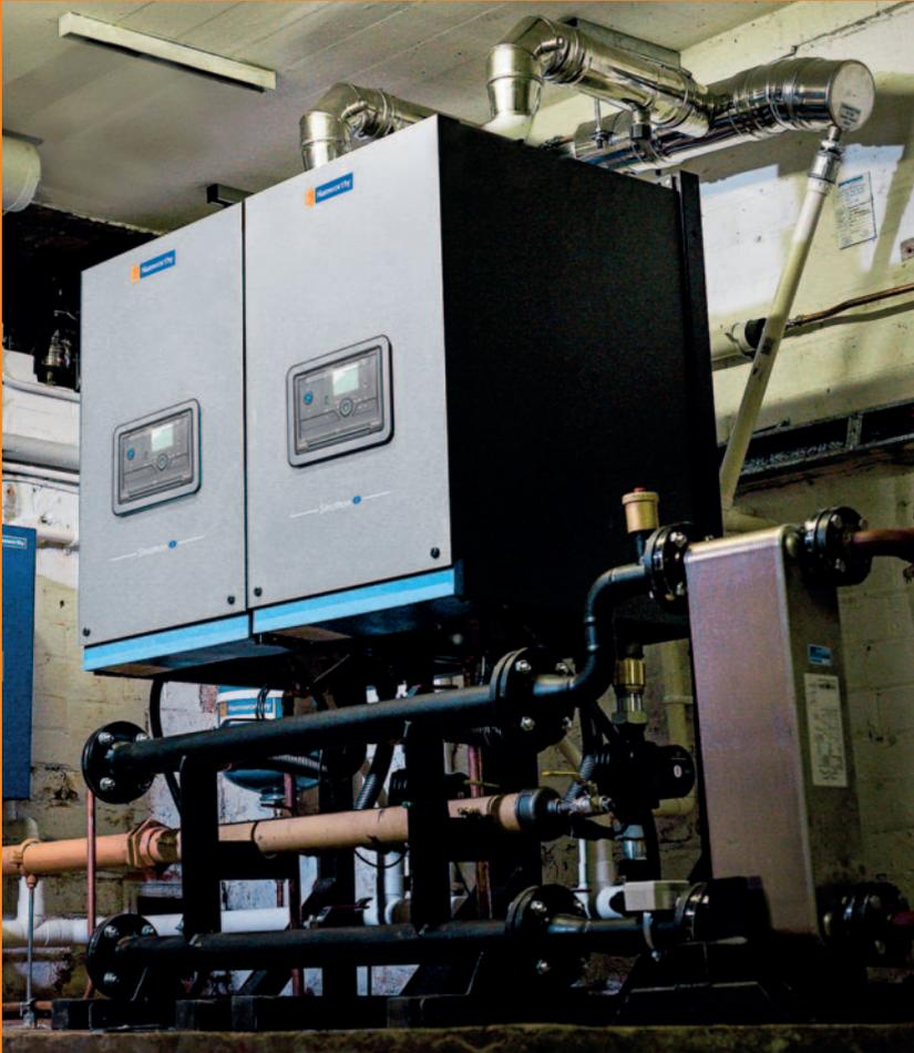
Our range of system separation plate heat exchangers are extremely compact and resilient with a gasket-free brazed design. They comprise of 316 stainless steel plates with copper brazing and are AHRI certified. Kits are supplied for connection straight onto the frame and header kit.
