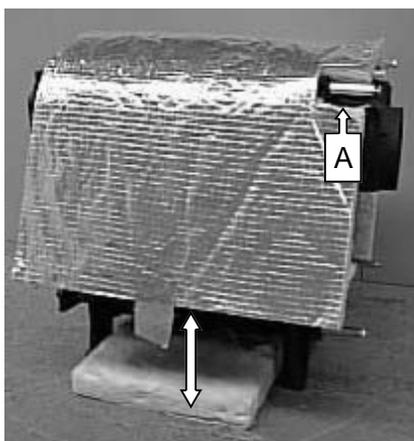
Wrap the insulation jacket around the boiler sections. Check that the cut outs (A) are positioned around the rear spacers and secure in position with duct tape.
