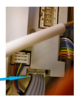
7 Fit the light grey plug to X2 on the AGU2.550A, no connection to this are required
