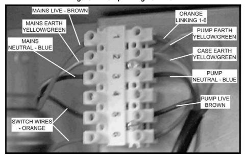
**Figure 24 Pump Wiring Terminal**
