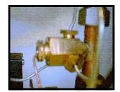
Figure 25 Capillary Nut
