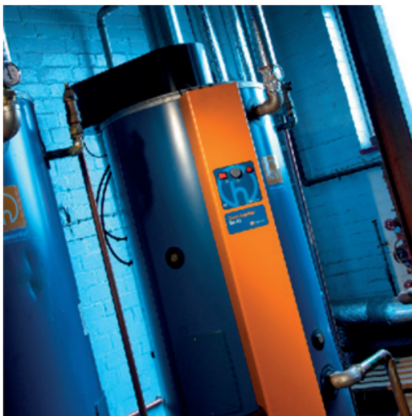
Dorchester DR-RS direct fired water heater in a typical plant room
