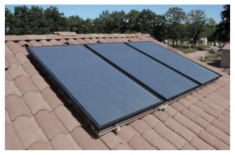
Single field array of three Trigon 2.3V vertical collectors, rail-mounted on a tiled sloping roof
