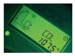
The Trigon standard and advanced solar controllers' principle function is very similar and relatively simple, i.e. it is the on/ off and speed control of the solar pump in the solar transfer station under differential temperature ( $\Delta T$ ), thermostat and timer control. The generic functions common to both controllers are described here with default settings taken from the standard controller and parameter names shown in italics.
