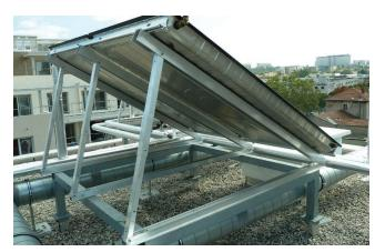
Trigon 2.3V collector array, flat roof mounted using a shallow A-Frame array fixing kit
