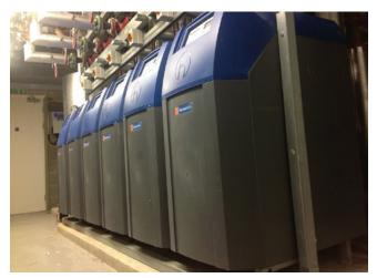
The Purewell Variheat condensing boilers have reduced **gas consumption by nearly 50%**. They provide the heating for the busy theatre as well as being the indirect primary heat source for the hot water via a Powerstock calorifier.
